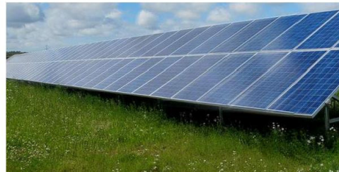
Benbole Solar Farm, Cornwall
