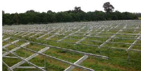
Frame structures prior to attachment of panels
